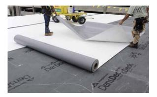
Independent ASTM D5635 puncture tests<sup>1</sup> indicated that thermoplastic membranes do not puncture as easily when 6.4 mm (<sup>1</sup>/<sub>4</sub> inch) DensDeck<sup>®</sup> Prime Roof Boards are used as a cover board, as compared to no cover board or high-density polyiso cover boards.
